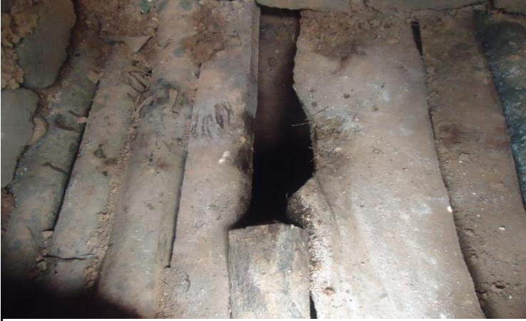
Cases were using non constructed and unroofed toilets
